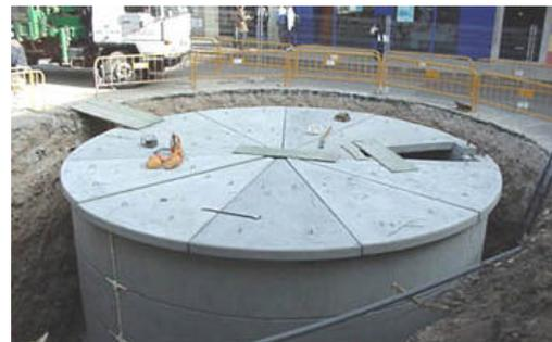
Top forged slab: prefabricated segments
