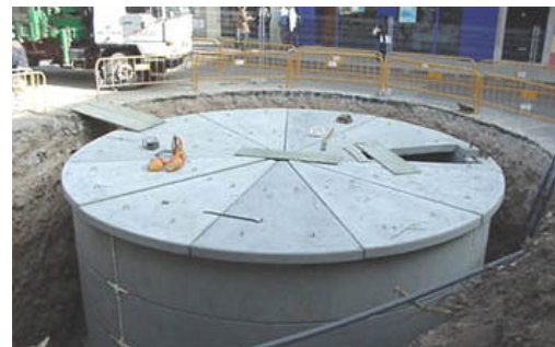
Top forged slab: prefabricated segments
